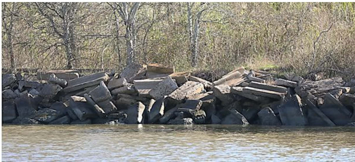
Figure 5-3 Typical Non-Engineered Shoreline of Pleasure Island
